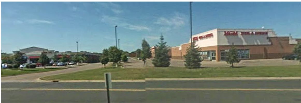
District 3, Maple Grove: Surrounding buildings and aerial within 500 feet of proposed facility:
